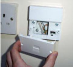
2. Plug your router or modem directly into this test socket via a microfilter.
